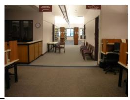
The interior finishes are in good to fair condition. Based on estimated Remaining Useful Life (RUL), the carpet and vinyl tile will require replacement during the assessment period. Interior painting and wall covering replacement will also be required during the assessment period. Wall covering replacement is relatively insignificant and can be done through routine maintenance.
